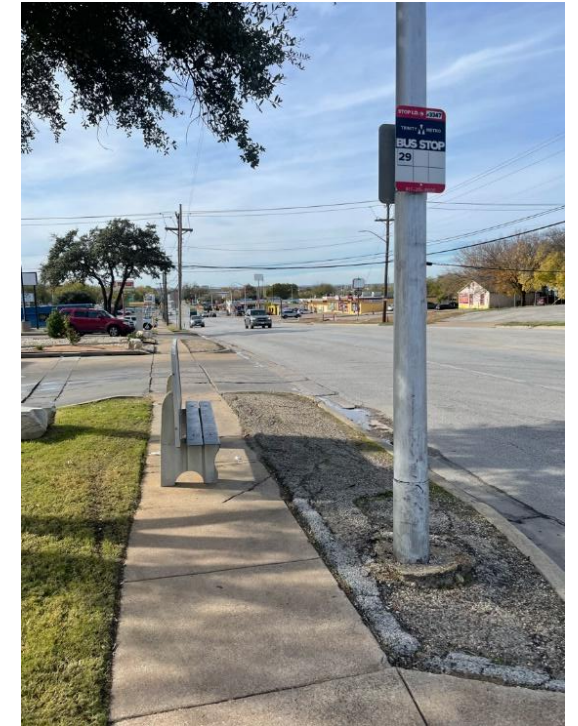
Bus Stop Bench Obstructing Sidewalk
