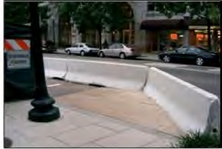
Figure 15. Proper separation devices must be used when diverting pedestrians into travel, parking, or bicycle lanes (Source: J. Barlow, Accessible Design for the Blind ; TTI)
