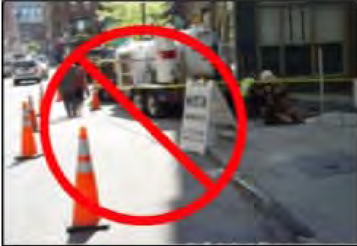
Figure 15. Proper separation devices must be used when diverting pedestrians into travel, parking, or bicycle lanes (Source: J. Barlow, Accessible Design for the Blind ; TTI)
